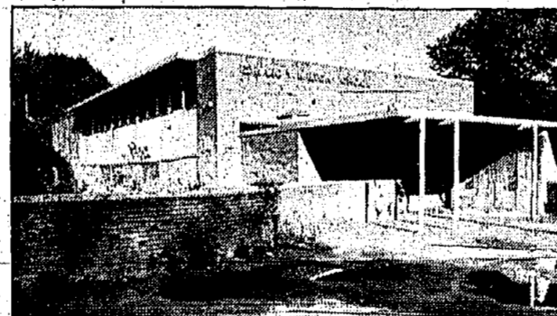
FUTURE DAY CARE CENTER — A portion of the old Edward V. Walton School building will soon be operated by the Summit Child Care Center Inc.
