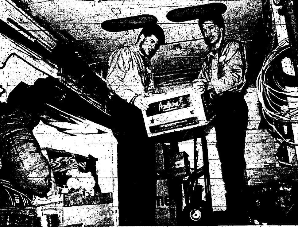
ON THE JOB — In their mobile workshop, Frank Londino, left, and Richard Worst of TRI Air Conditioning prepare to install a humidifier.
