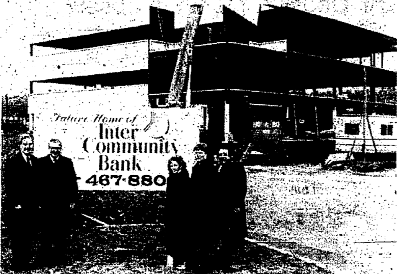
GOING UP — At the construction site of Inter Community Bank's newest office in Springfield are, left to right, Jerome Waldor, bank chairman; Nazario Paragano, bancorp chairman; Denise Casale, branch manager; Mark Fogt, president and chief executive officer; and Michael Bono, senior vice president, sales and marketing.
