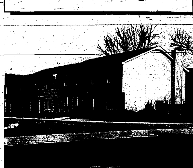
RIVER'S EDGE, a new townhome community, is located at 833 Valley St. in Union.
