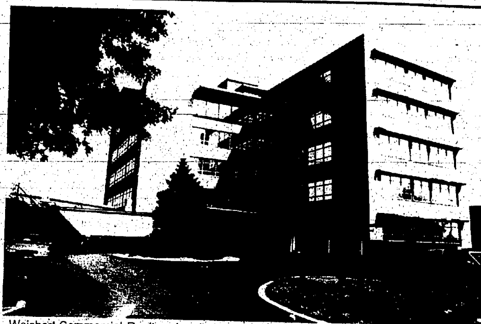
Weichert Commercial Realtors has been selected to market this 100,000-square-foot office complex on Park Avenue in Linden.
