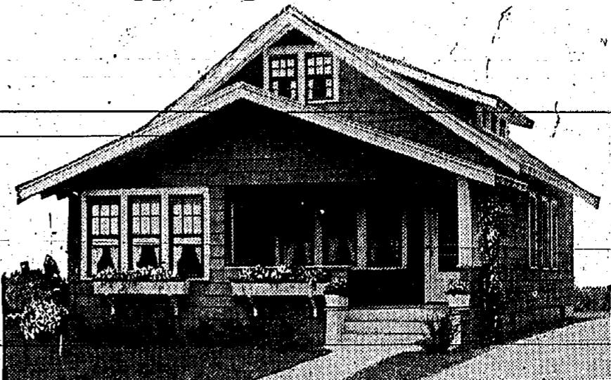
Shingles have been used effectively on the walls of this five-room bungalow. The unusual lines of the gable in the porch roof and the well-balanced windows make the exterior attractive. The house is 24 feet by 34 feet.
