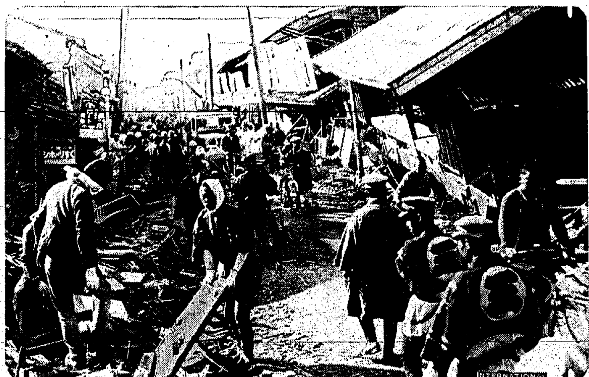
Street scene in Miblan, Japan, after the recent earthquake. A number of persons were killed in this town and many houses were destroyed.
