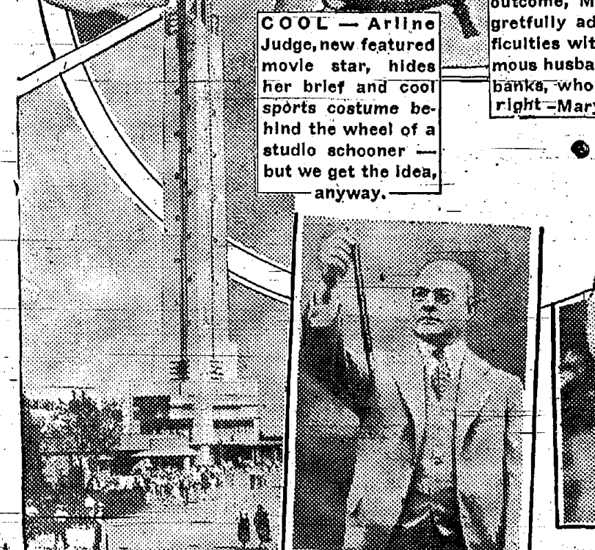
TEST GIANT THERMOMETER—C. A. Donnel, senior meteorologist of the U. S. weather bureau in Chicago, compares the reading on his official "sling" thermometer with the 2-foot wide "mercury" columns on the huge Havoline thermometer shown in the background. The 218-foot tower, the largest thermometer in the world, shows visitors to the Century of Progress Exposition just how hot it is day and night.
