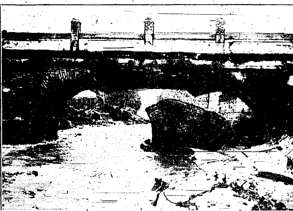
IN WAKE OF STORM FATAL TO THOUSANDS —A bridge wrecked in the terrific hurricane that recently struck El Salvador, bringing death to thousands in the little Central American republic and causing millions of dollars of damage. The force of the storm can be seen from this picture, which shows the heavy under-structure of the bridge completely torn away.
