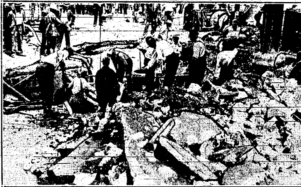
GEYSER OPENS STREET —When a 48-inch water main burst in Brooklyn, N. Y., it ripped up the pavement and poured thousands of gallons of water into basements in the neighborhood. Householders went without water when the supply had to be shut off. Here are workmen avoiding a tangle of cables as they start repairs.
