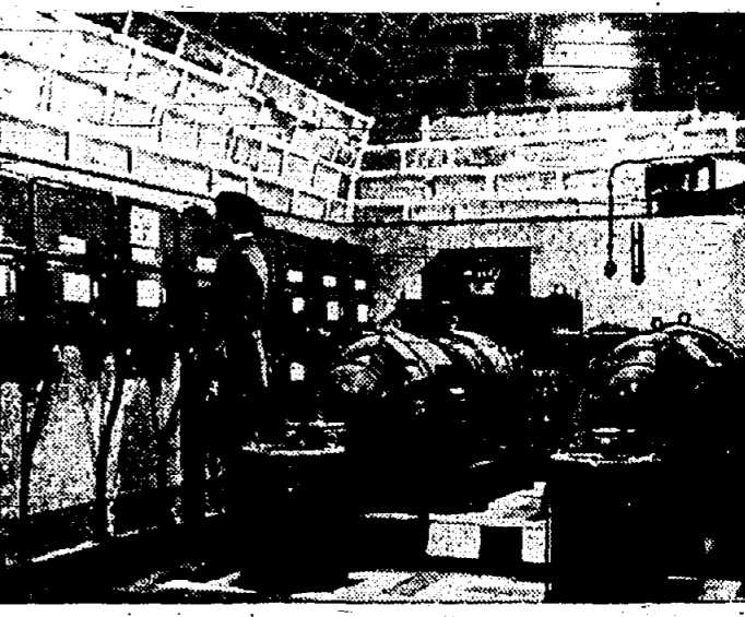
MAGINOT LINE—Older, more scientifically constructed, this series of "underground battalions" can probably be manned with less difficulty than the newer West Wall. Photo shows officer operating underground power plant in one of the fortresses.
