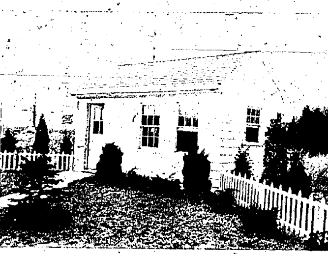
Field office of Anshore Home Builders, Henshaw and Mountain avenues, which has been temporarily along to the local Boy Scout Troop 66 for its headquarters by Harry Tzessis, owner.
