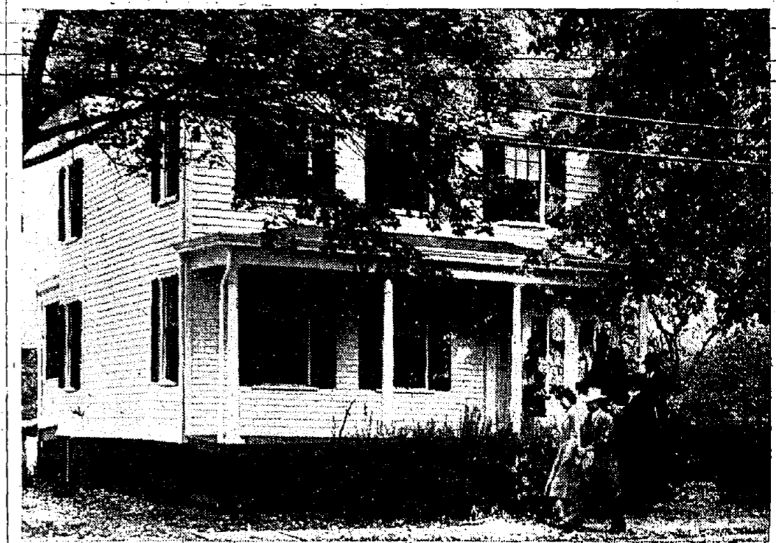
Exterior view of the redecorated former Sarah A. Bailey House in Main street, bequeathed to the township as a municipal library. Walking on the sidewalk in front of the building may be seen Mrs. Nicholas C. Schmidt, library president, and Fred A. Ebsasser, architect. On the steps are Mrs. Ralph H. Tittle, trustee, and Mayor Wilbur M. Selander, and on the porch are Mrs. Charles T. Smith, trustee, and Valfrid Palmer, contractor. Photo by William Zimmerman
