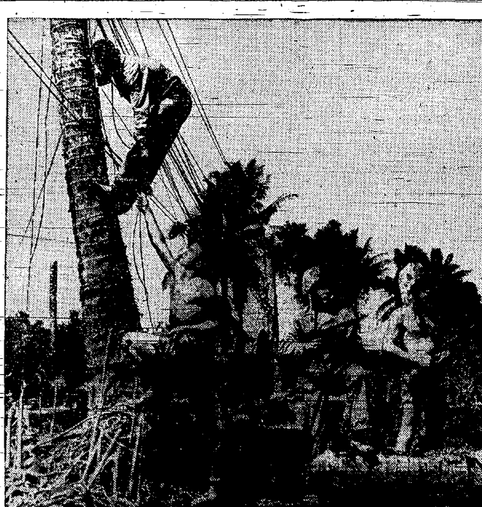
U. S. Marines in the South Pacific use palm trees for telephone poles as they string communication lines.
