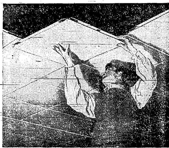
CEILING PANELS IN THE house are installed with air spaces between panels and insulation layer, through which hot air moves to heat room.
