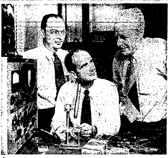
WITH THIS APPARATUS some of the first investigations leading to the discovery of the Transistor, a tiny gadget which will perform almost all the functions of a vacuum tube, were made.
