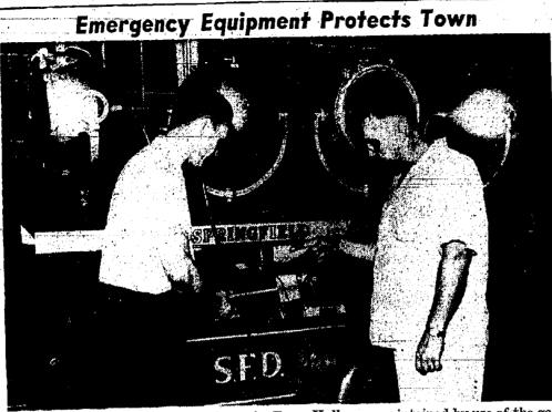
Police radio, lights and machinery in Town Hall were maintained by use of the gasoline-driven municipal power unit during four-hour electric current failure last week. Shown examining voltage regulator on emergency generator are Firemen Ormond Mesker ment this year. Average enrolland Charles Schilling, left to right. Break in main line of Jersey Central Power and Light Company caused the light failure. It was attributed to the heat wave.
