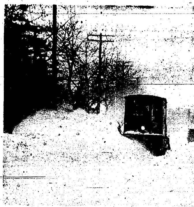
WHEN WEATHER reports forecast snow for suburban areas, county highway departments swing into action with their snow fighting machines to keep the highways clear for moving traffic. Above, a plow sends a plume of snow from the right of way.
