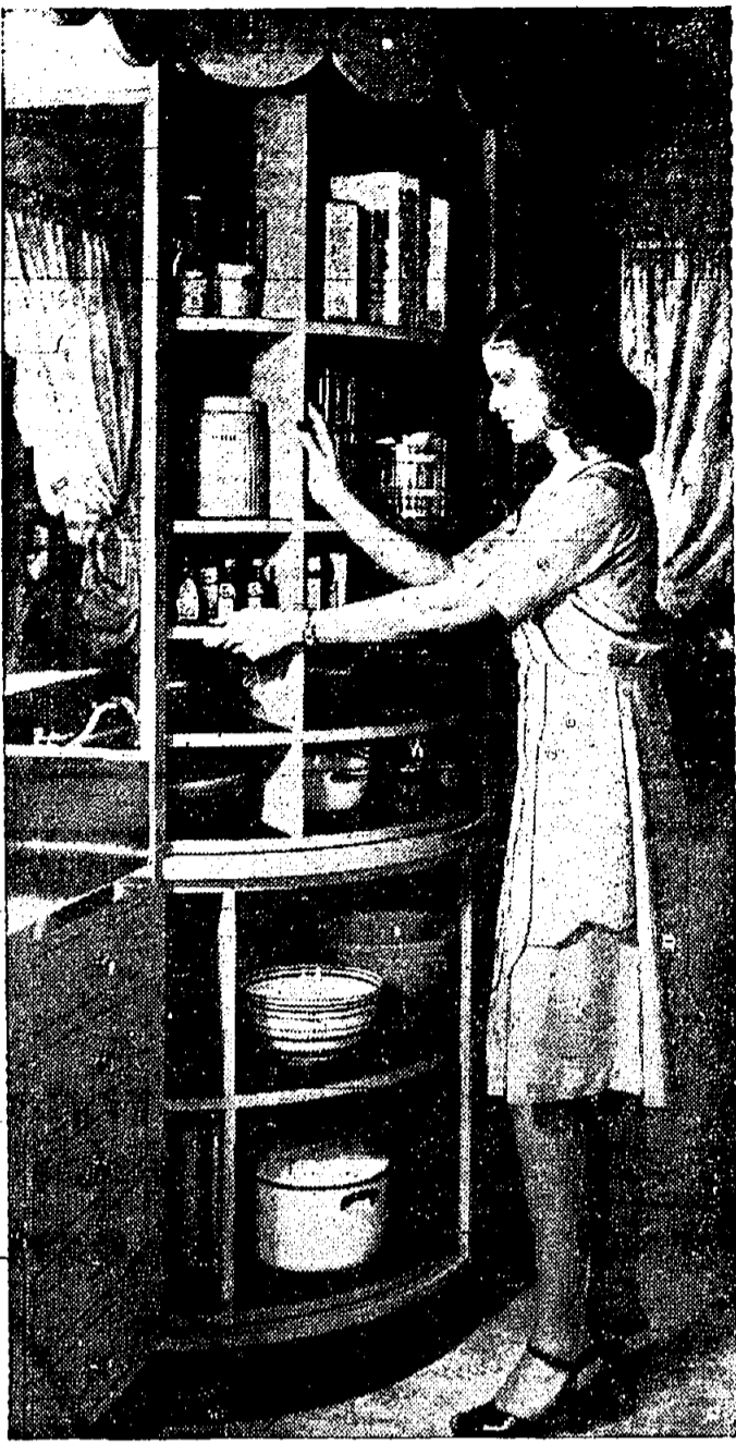
KITCHEN REMODELING proved to be a popular pastime among housewives last year. Among the tricks learned were that a counter height of 38 to 40 inches was the most practical. In some kitchens revolving shelves were installed allowing greater visibility of stored supplies.
