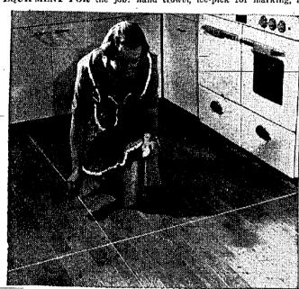
LOCATE THE EXACT center of the floor and mark it off with chalk working base or starting point for laying the tiles.
