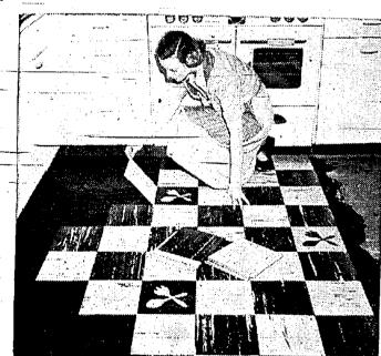
REPEAT ABOVE process for other half of floor; work from center toward wall containing a door opening so you can leave the room.
