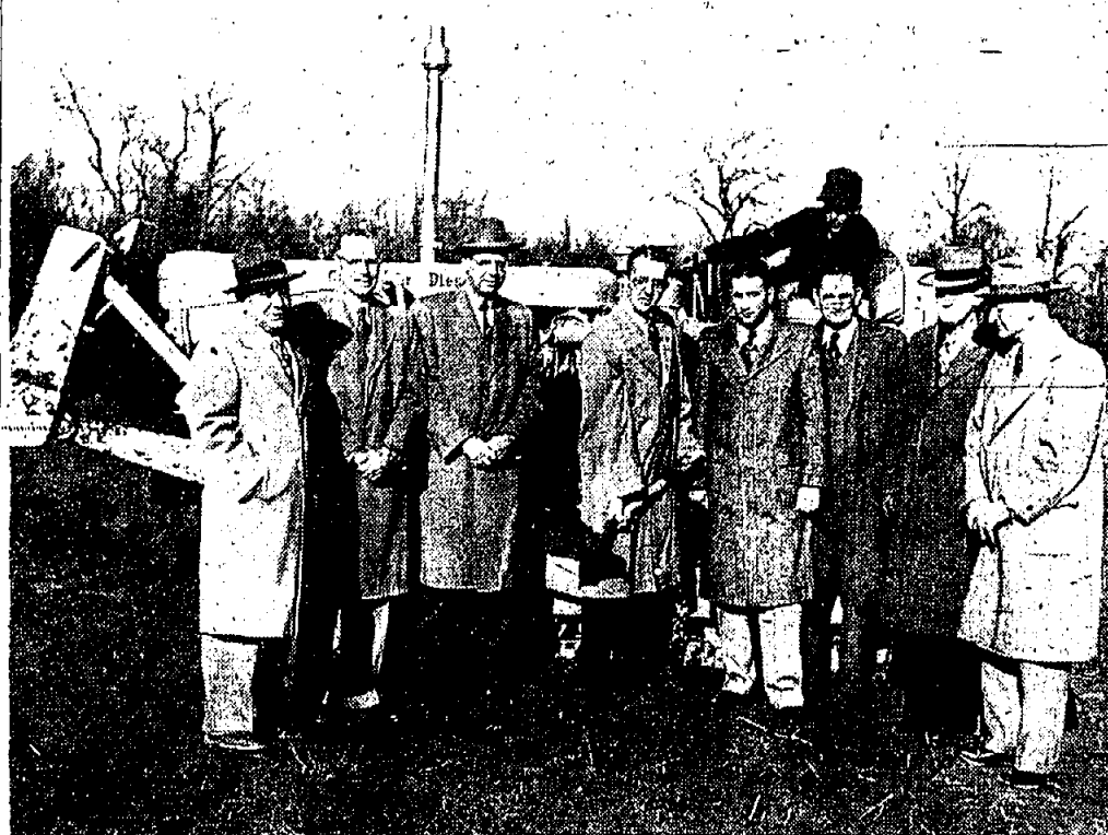
School system and township officials participate in the ceremony marking the launching of construction for the $800,000 upper grades school in South Springfield avenue...
