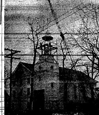
CLOSING THE TOWER-Crane shown lowering the cupola to the new tower after church bell was put in place on the remodeled Methodist Church.
