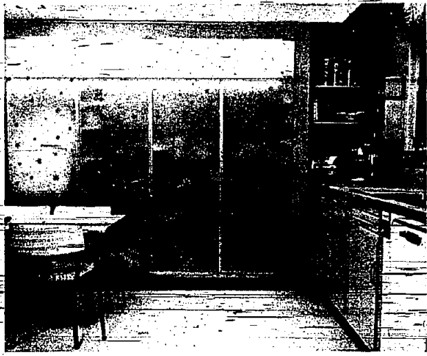
The new storage cupboard runs the full width of the room. Doors are fibre-glass panels made to slide on nylon rollers. Inside lights suffuse the surface with a soft glow.
