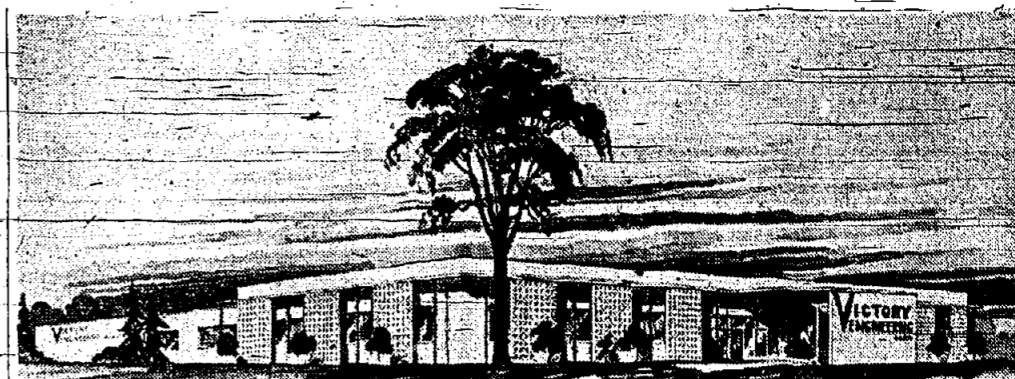
NEW BUILDING FOR VICTORY ENGINEER—when completed, new factory will facilitate production...
