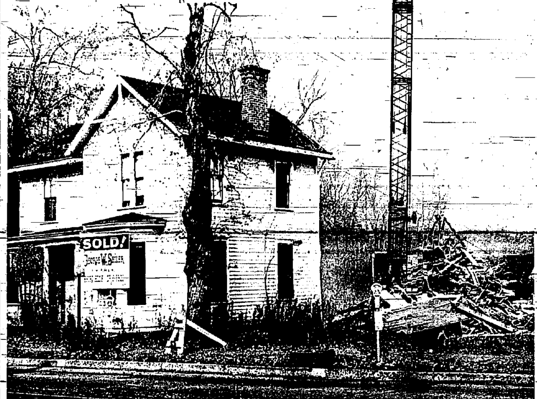
END OF A LANDMARK--House at 294 Morris Avenue, presumed to be about 140 years old came down last week to make way for a new office building to be located on the site. The house, originally owned by the Sickley family, one of Springfield's oldest, was purchased in June of 1925 by Richard Bunnell of Bunnell Bros. Insurance Co. of Springfield. The Bunnells lived there until 1959. In its earlier days, the house doubled as a tavern. More recently an addition was put on the back section. Pictured on the left is the bulldozer starting its work on the rear of the structure, while the photo on the right depicts the house in its prime.
