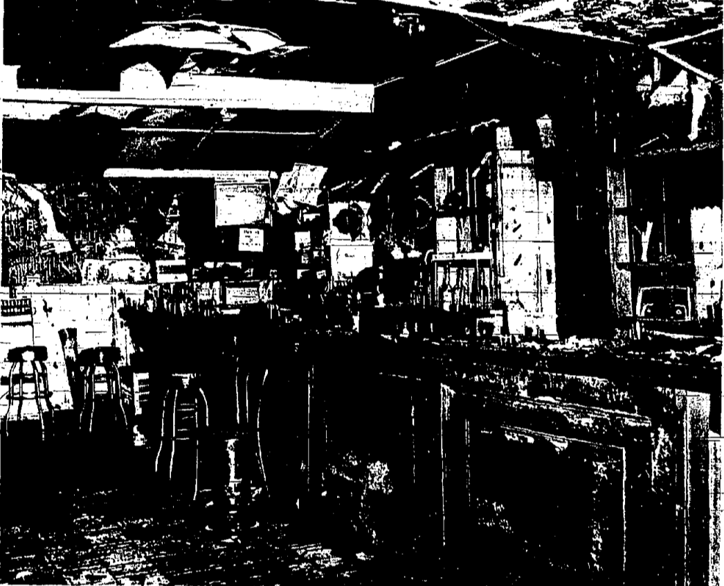
INSIDE VIEW—Pictured above is all that remained after Evergreen fire. Fire damage was mostly contained to the bar area of the popular lodge. Workmen spent all Thursday night patching up ceiling which was completely burned out.
