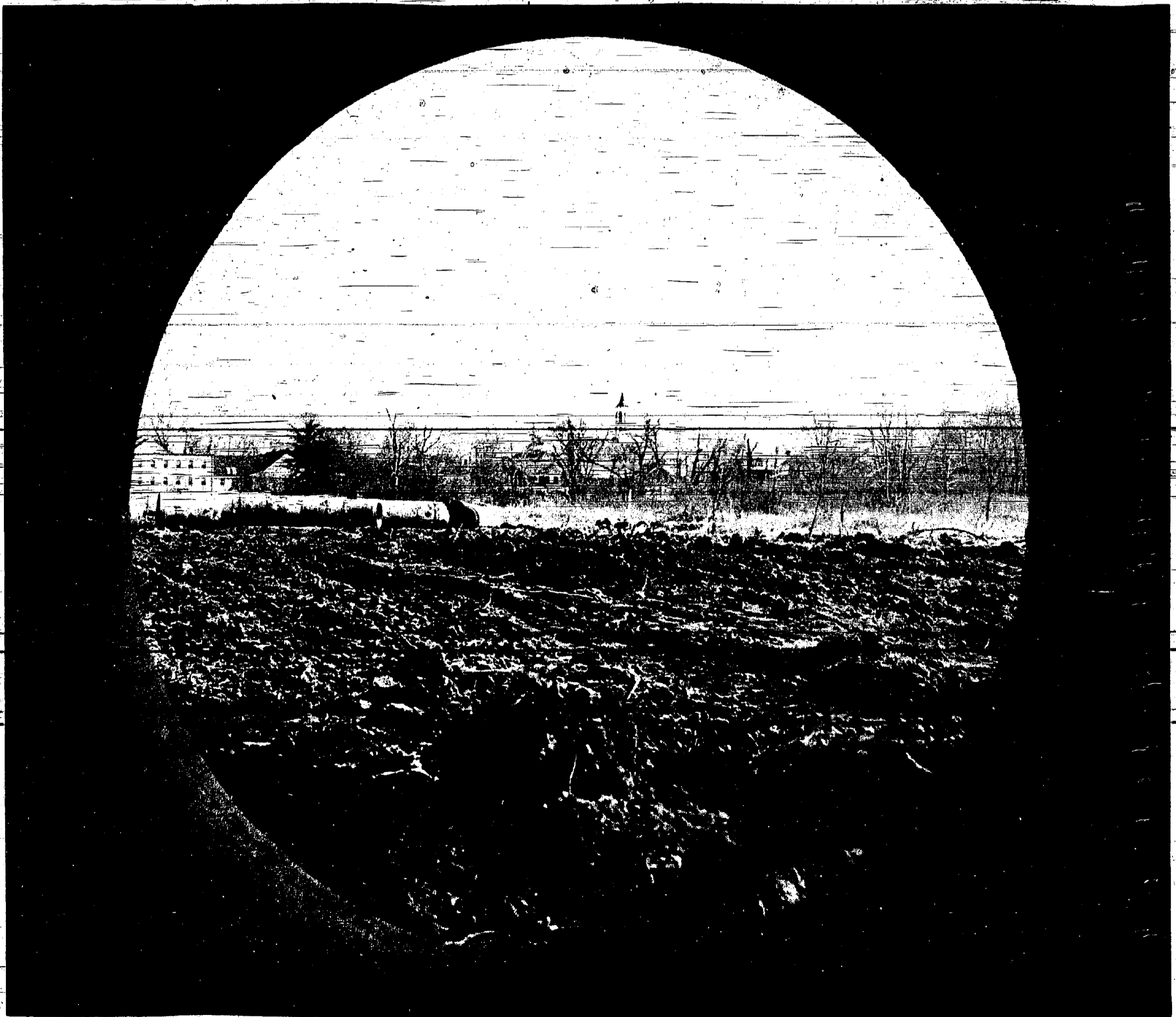
SPRINGFIELD MUNICIPAL SWIMMING POOL SITE BEING CLEARED: As seen through the camera lens of Fred Keesing.
