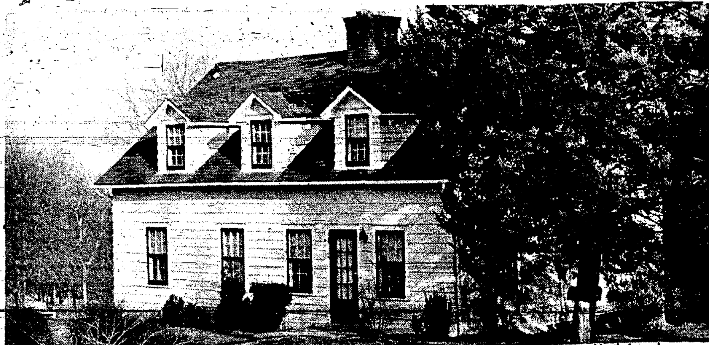
THE BALTUS ROLL HOUSE as it looks now, with dormers in the roof, installed by the previous owner. The house is just over the Springfield-Mountainside boundary, in Mountainside. It is owned by the Misses Edna and Ethel Clements. (Photo by Stewart C. Fulton)
