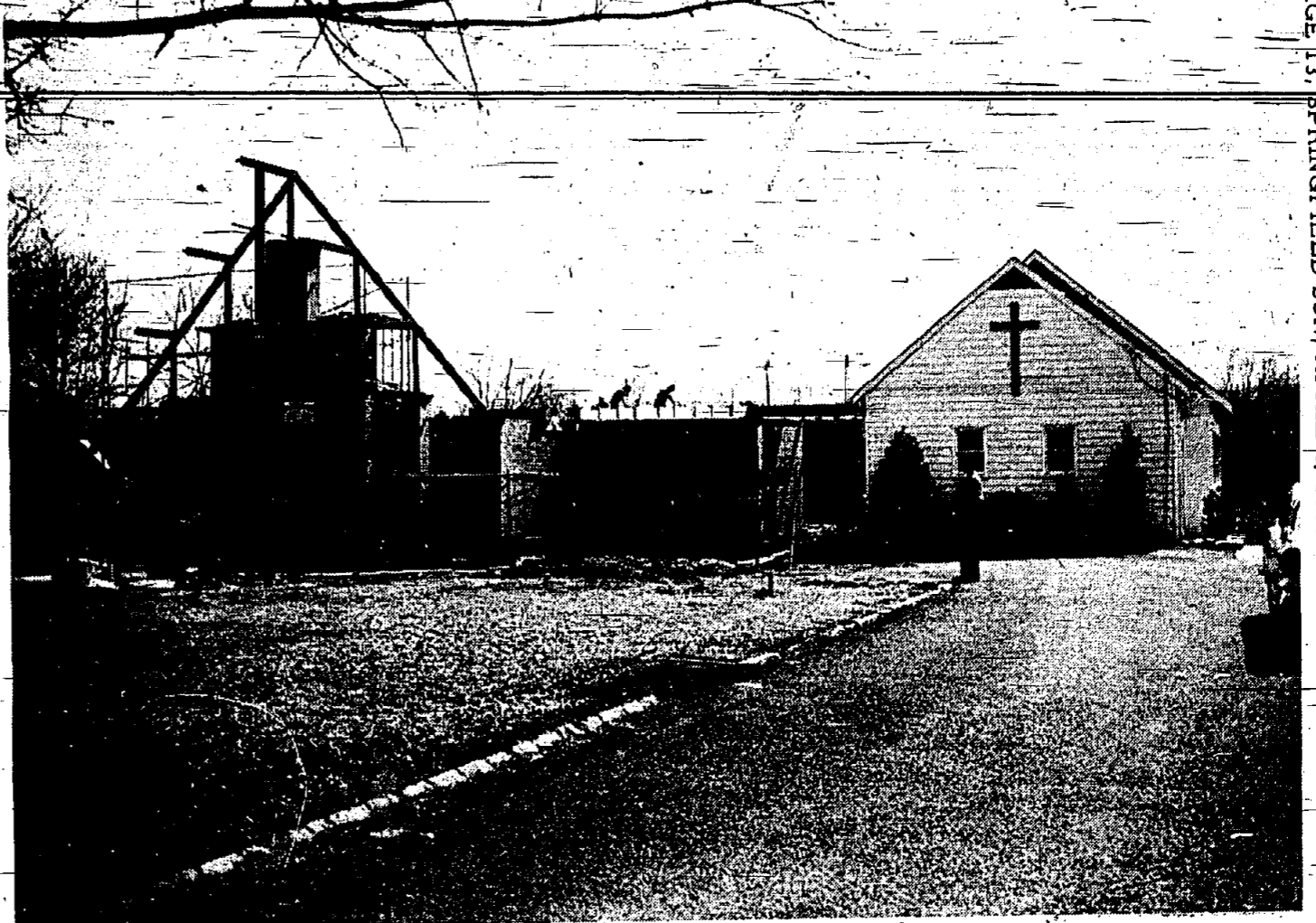
SHOWN VIEWING construction at the new Holy Cross Lutheran Church, 639 Mountain Avenue, Springfield, is the Pastor, Lester Messerschmidt. Ground was broken for the $131,000 structure on October 7, 1962. Completion is slated for late summer of this year.
