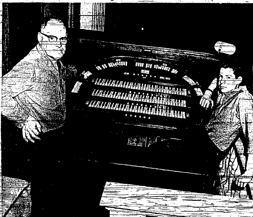
ADMIRING HANDIWORK - Howard Day and son Allan take a pause from their labor of love, the restoration and overhaul of an old pipe organ that has seen its better days down at the Masonic Temple in Elizabeth. Photo by Daron Studio
