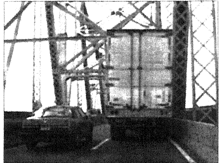
The narrow Goethals Bridge, which connects New Jersey to Staten Island, N.Y., may soon be replaced by an entirely new structure.
