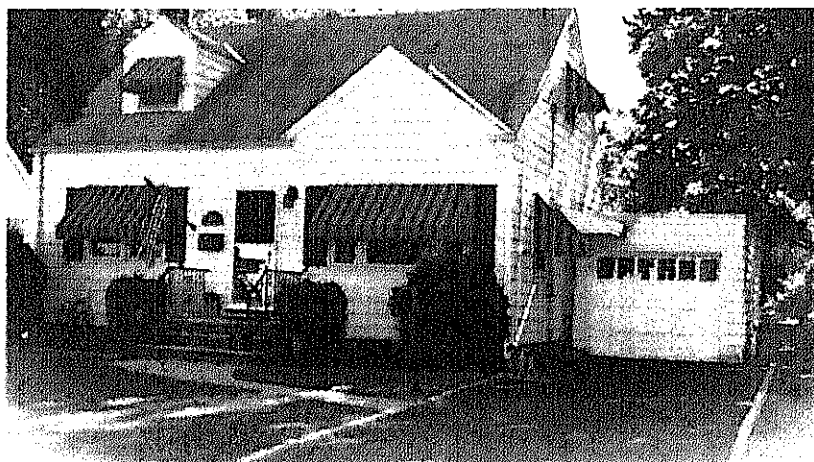
Owners of this Union County home owed more than $390,000 on their mortgage and were able to avoid foreclosure by short-selling the property for $256,000 with the assistance of Striker Realty in Linden.
