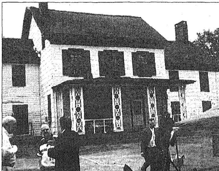
Above, the 250-year-old Homestead Farm at the newly-christened Oak Ridge Park in Clark will be restored using historic preservation grant funding. Below, the former golf course is being transformed into a county park.
