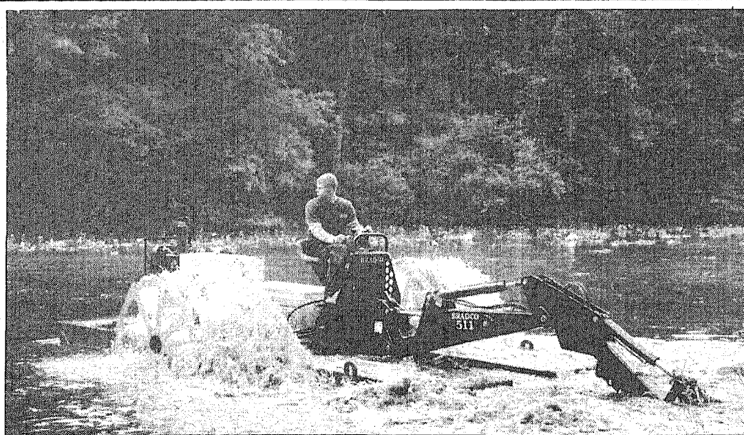
IT'S NO SURPRISE — With the sidewheels churning in reverse, Kyle Keane of Port Jervis, N.Y., drags the hydro-rake along the bottom of Lake Surprise in Union County's Watchung Reservation in order to dig the roots of the spatterdock, the lily pad species that had taken over the eastern end of the lake.
