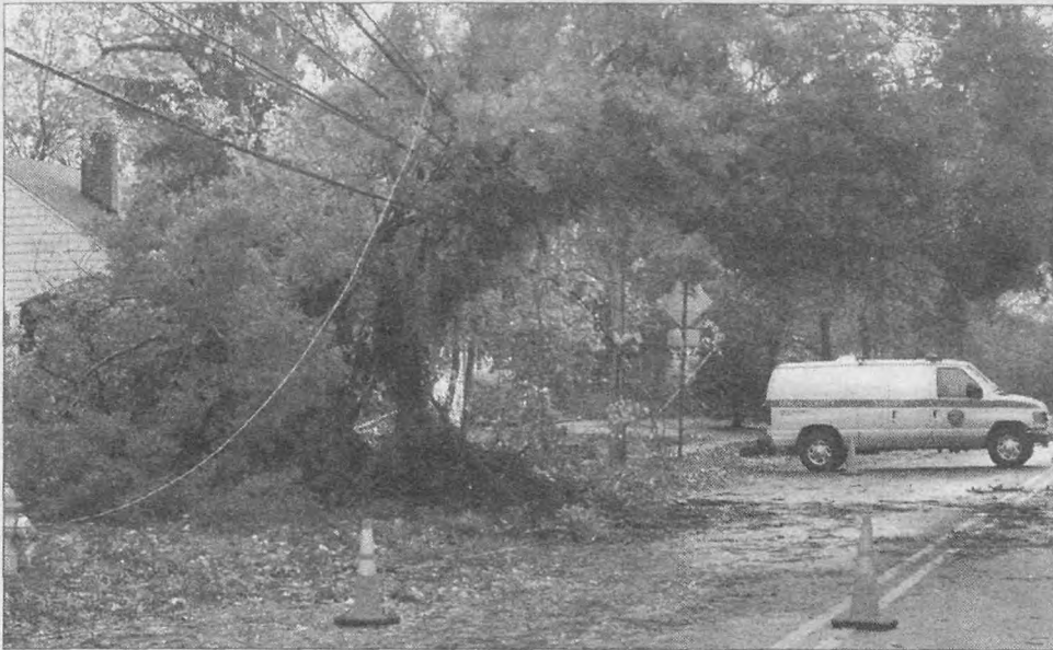
Photo Courtesy of Jim Lowney/County of Union
